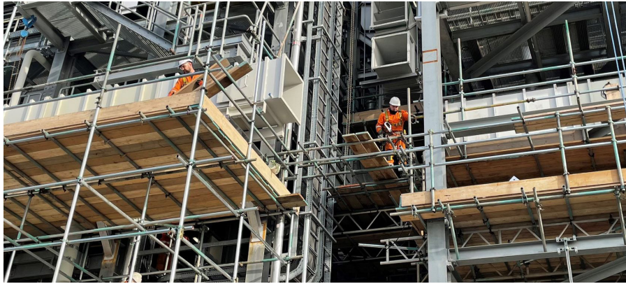
New oFGR ducting being fitted to the outside of the plant
