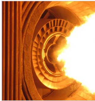
RJM Ultra-Low NO x Burner for wall-fired boilers
