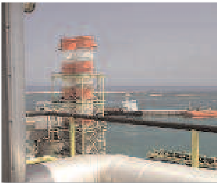
Figure 1. The Brindisi plant
